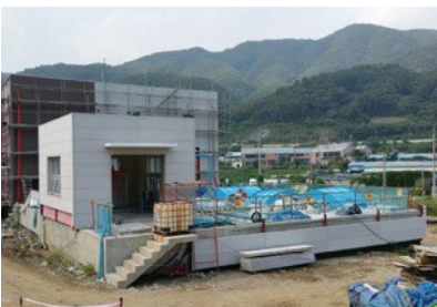
HADO WWTP | 16.4 MGD February 2017
